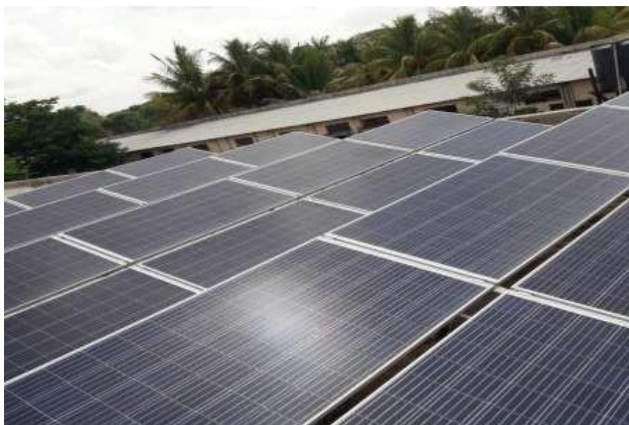
Installation of Solar Power plant on rooftop
