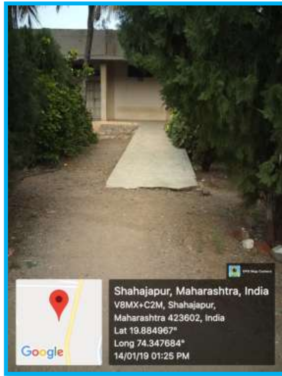
Divyangjan friendly Ramp
