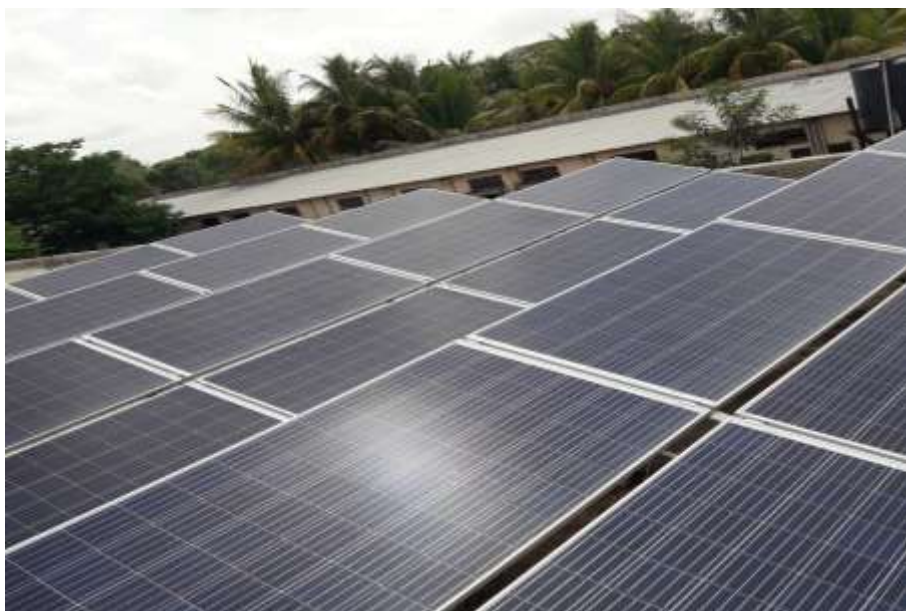
Installation of Solar Power plant on rooftop
